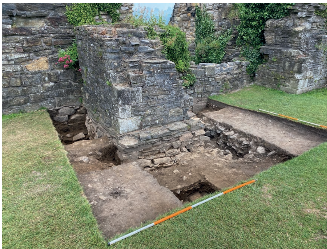
Figure 3. Overall view of Trench 1. The gap in the curtain wall is visible with the Ministry of Works wall infilling the gap. The difference between the medieval walling and the Ministry-created 'buttress' is also clear. Finally, the loosely compacted rubble fill of the former sally port ramp can be seen in section in the right-hand side of the trench
